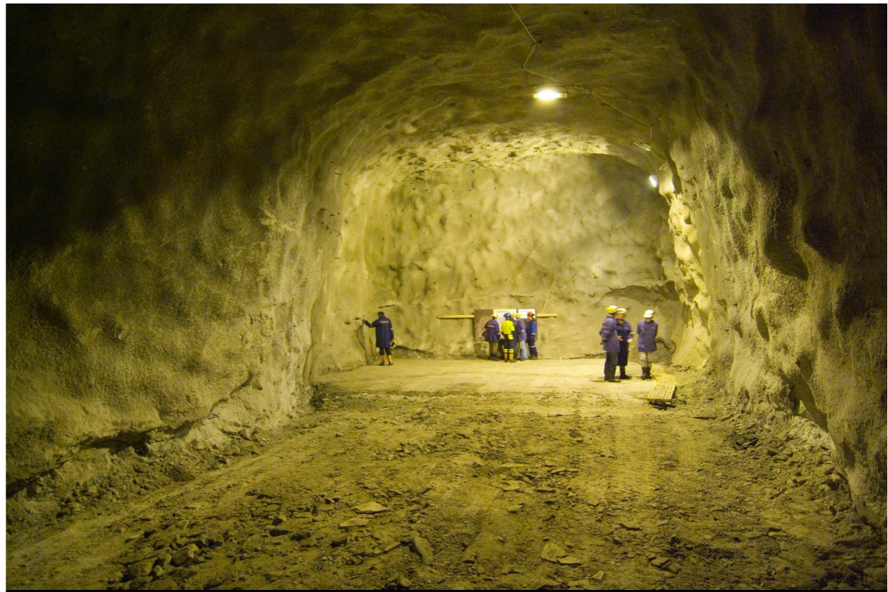
250 m long tunnel and a cavern at 1400m excavated for LAGUNA R&D
